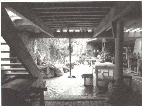
The Garden of the communal space for exchanging 'techno-playful' knowledge, under-construction
